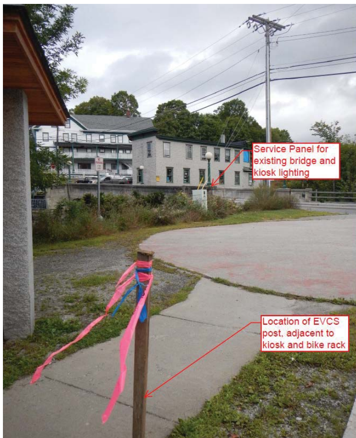
Looking NW from EVCS location stake toward service panel and Main Street Bridge
