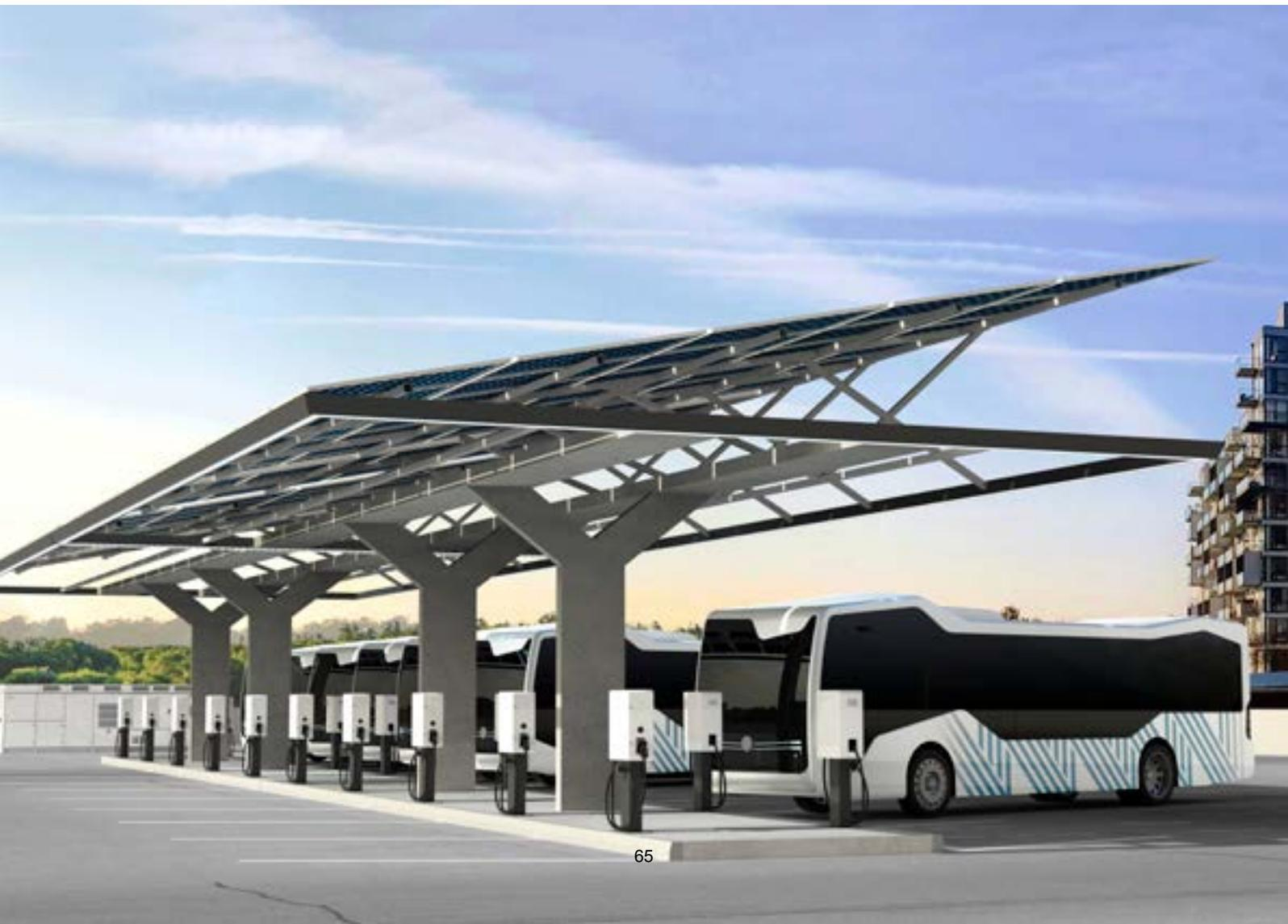
NBi Station allows the EV charging from different power sources: photovoltaic field, battery system and utility grid.
